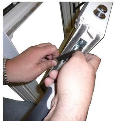
Depress retaining clip to allow restrictor arm to be disengaged
