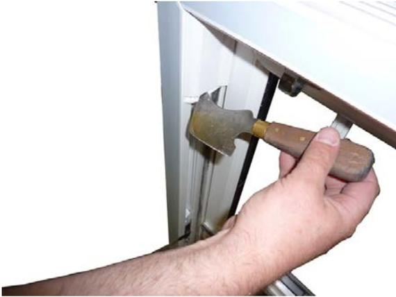
Carefully remove the end cover cap from the frame stop taking care not to damage the frame or sash stop
