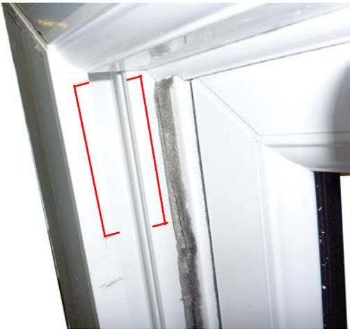
From both sides of the retaining groove measure back 5mm and mark the frame
