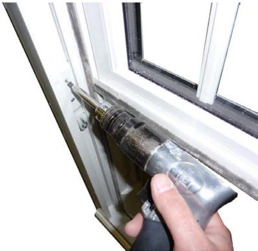
Remove the screws securing the springs
