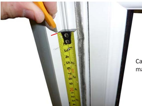
Carefully measure 20mm up from the pencil line and mark the outer frame
