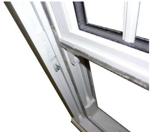
Once all the screws have been removed slide the spring assembly to the top of the frame and remove by sliding the assembly through the aperture that has been made in the frame, remove the damaged shoe through the same aperture and replace
