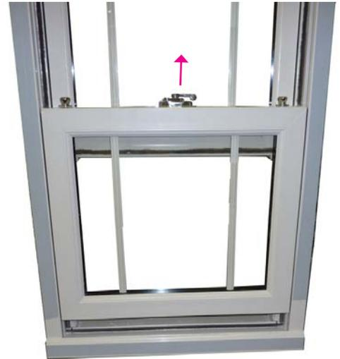
Slide the sash upwards to clear the internal rebate
