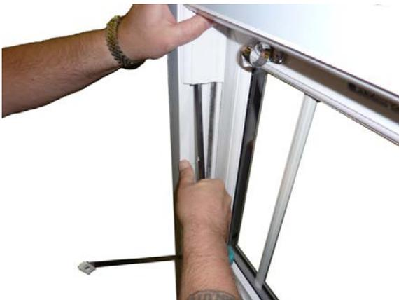
Use a screwdriver or similar to carefully prise the clip fit sash stop from its location groove.
