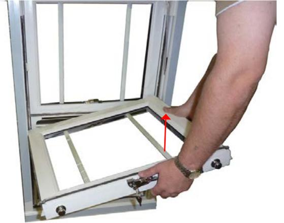
Once one side of the sash has been disengaged from the shoe this will then allow the other side of the sash to also be disengaged and the sash removed.
