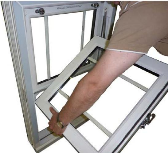
Once the sash is removed it should be possible to determine which shoe is damaged and requires replacing
