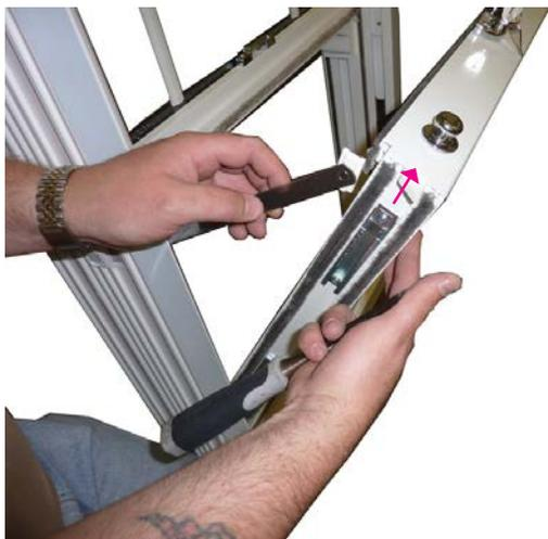
Slide restrictor arm upwards to remove from channel.
