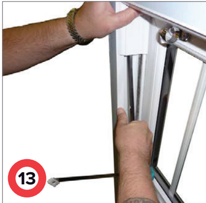
13 Use a screwdriver or similar to carefully prise the clip fit sash stop from its location groove.
