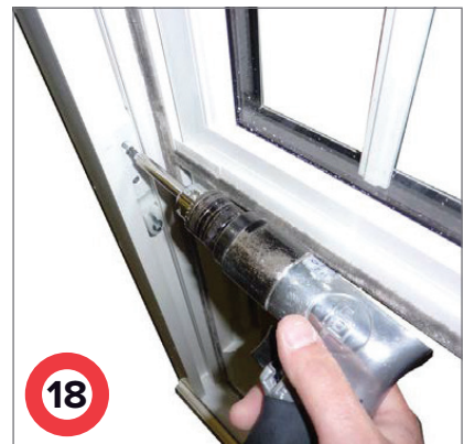
18 Remove the screws securing the springs.
