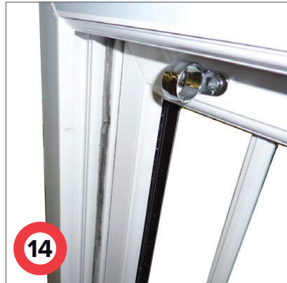
14 The retaining groove for the coil springs and shoe is now clearly visible.
