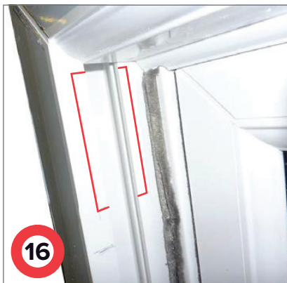
16 From both sides of the retaining groove measure back 5mm and mark the frame.
