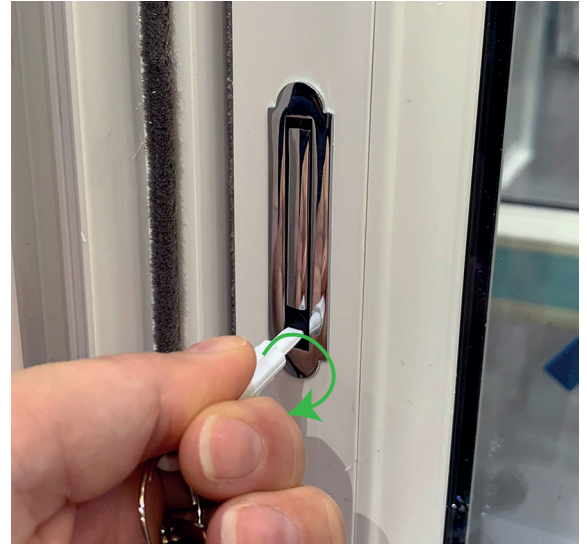
Fit key into cam and turn clockwise to open restrictor
