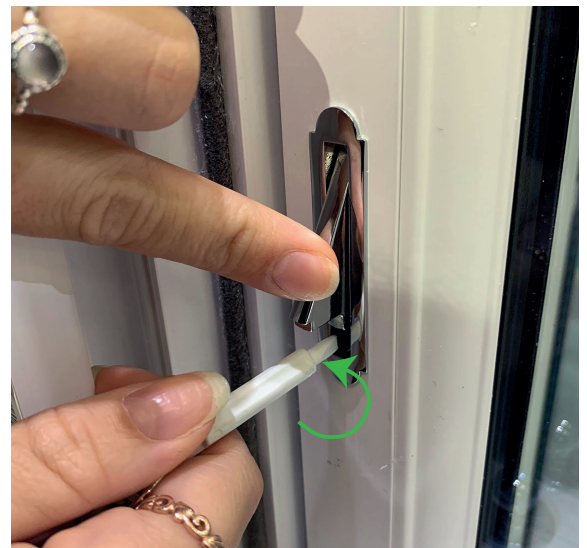
Push restrictor in and turn cam anti clockwise to close/lock restrictor
